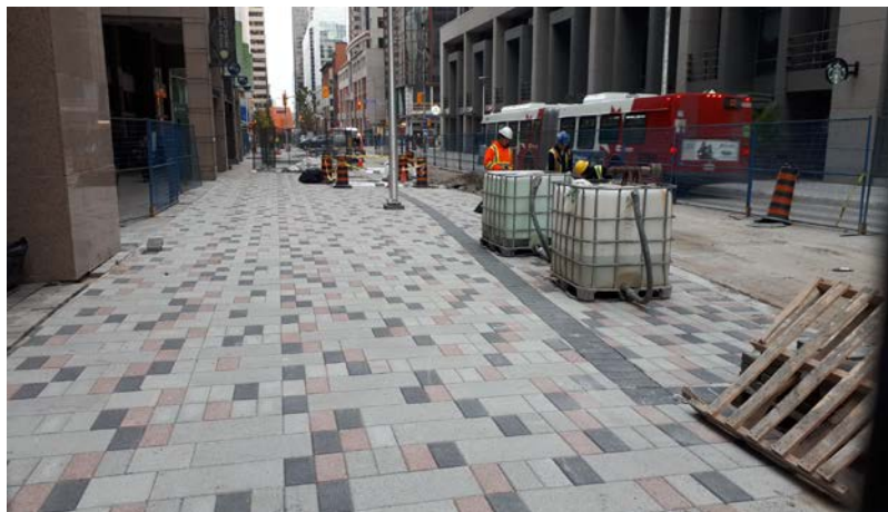
Queen Street Streetscaping Project
