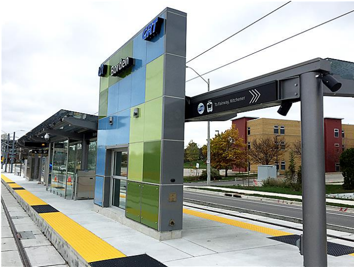
Waterloo Stage 1 LRT
