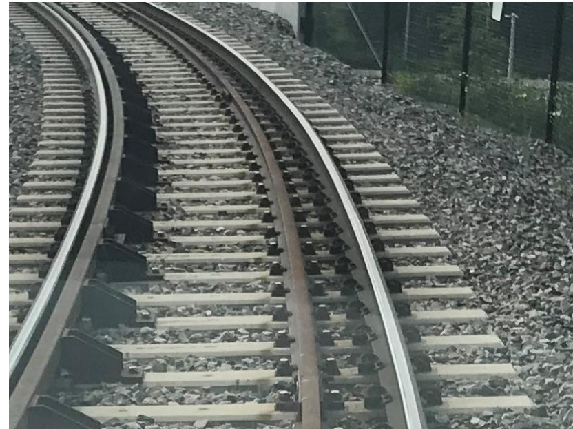
Fig. 1 welded track (above)
