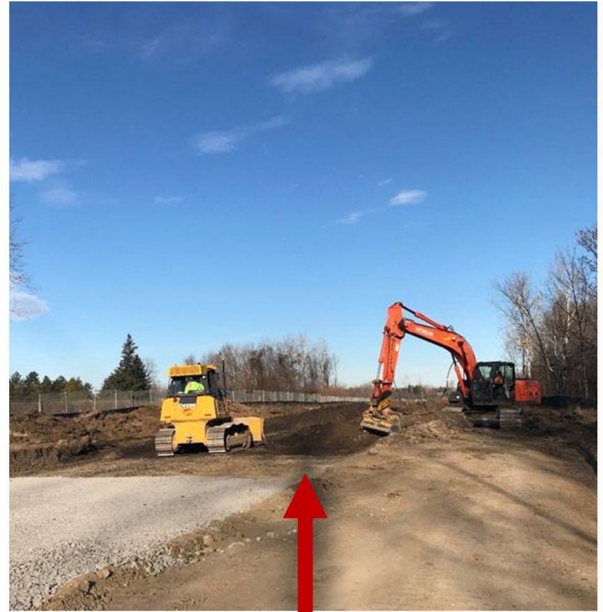
Stripping and capping between Lester and Leitrim
