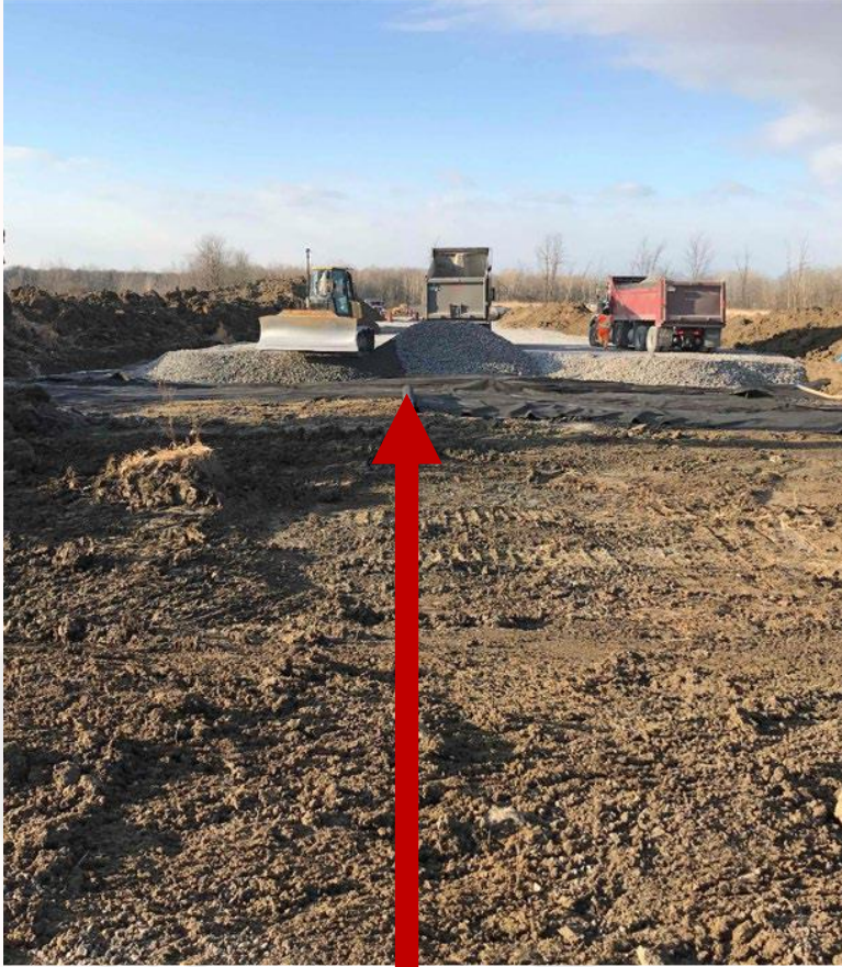
Stripping and capping between Bowesville and Limebank
