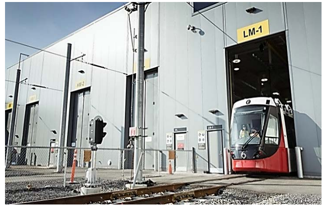
Testing at Belfast Yard
