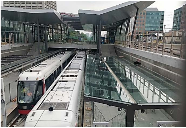
LRV Testing at Tunney's Pasture
